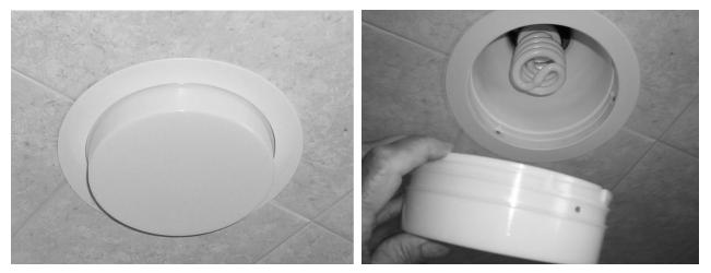
break something. The plastic globe turns counterclockwise about 1/8 of a turn. There is a tab in the metal part of the fixture that aligns with the slot in the plastic globe. If it doesn't seem to want to move, press on the bezel with one hand while turning the globe with the other and then pull it down. Now you can change the bulb and clean the fixture.
