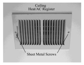
When reinstalling, align the screws in the respective holes in the sheet metal behind the vent without holding it flush to the ceiling. This will make it easier to find and or see where they are supposed to go.
