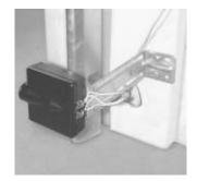
sensor isn't working, the door won't work, either. If a problem exists with the safety eyes that are preventing the door from closing, and you know nothing is in the way, the door can be closed by holding the wall control button in until the door is fully closed. (The remote control will not work.)
